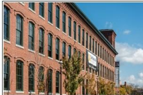
The Counting House Apartments in Lowell opened earlier this year and has rented 50 of its 52 units.
